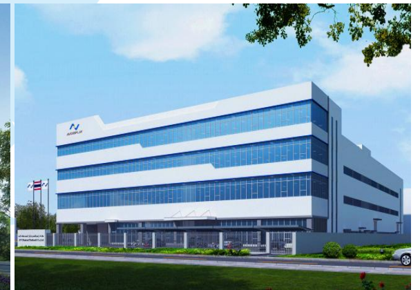
Thailand Factory (under construction)
