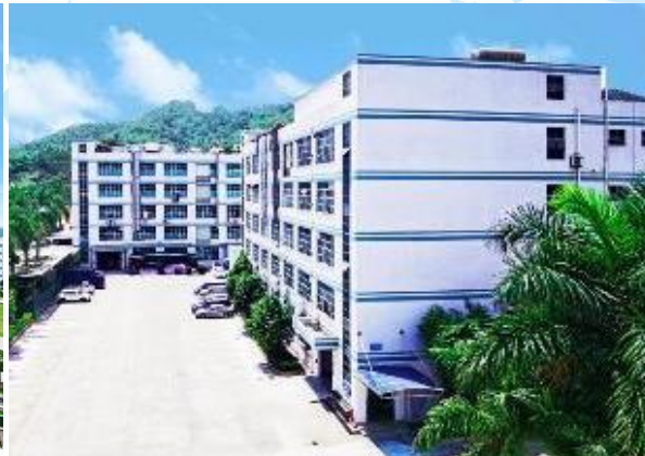
Shenzhen Headquarter & Factory
