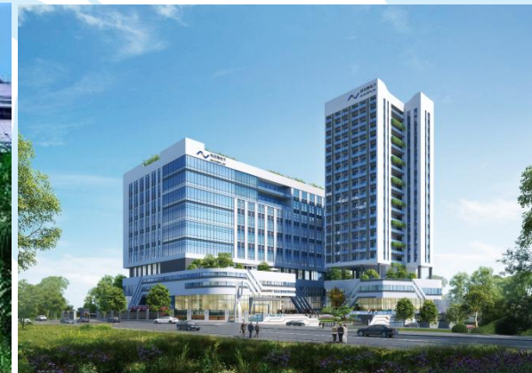
Shenzhen New Industrial Park (under construction)
